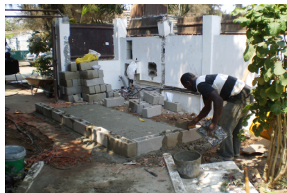
The plinth being laid for the new standby generator
